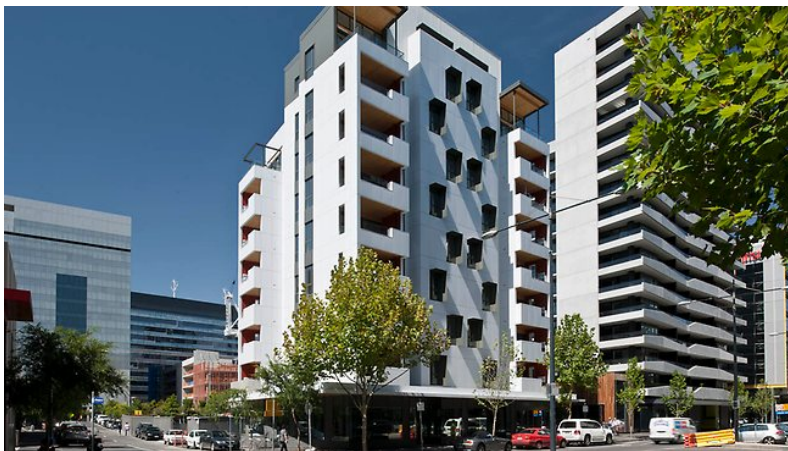
The Forté Tower in Melbourne, Australia, which is the largest modern apartment building in the world built of wood and makes extensive use of cross laminated timber (CLT). Photo credit: Lend Lease.
